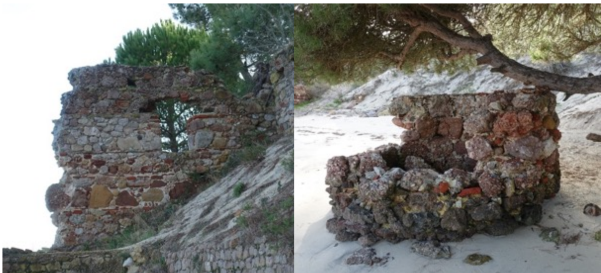
Figure 5: Wall with window in workshop 21 (left) and well in workshop 23 (right).
