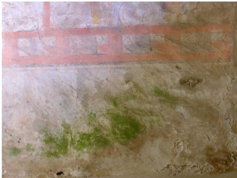
Figure 9: Algae in Wall c in the Tróia Basilica, before biocide application.
