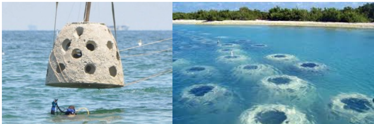
Figure 8: Examples of reef ball systems deployed in Italy. Sources: www.ilrestodelcarlino.it (left); www.reefballitalia.it (right).
